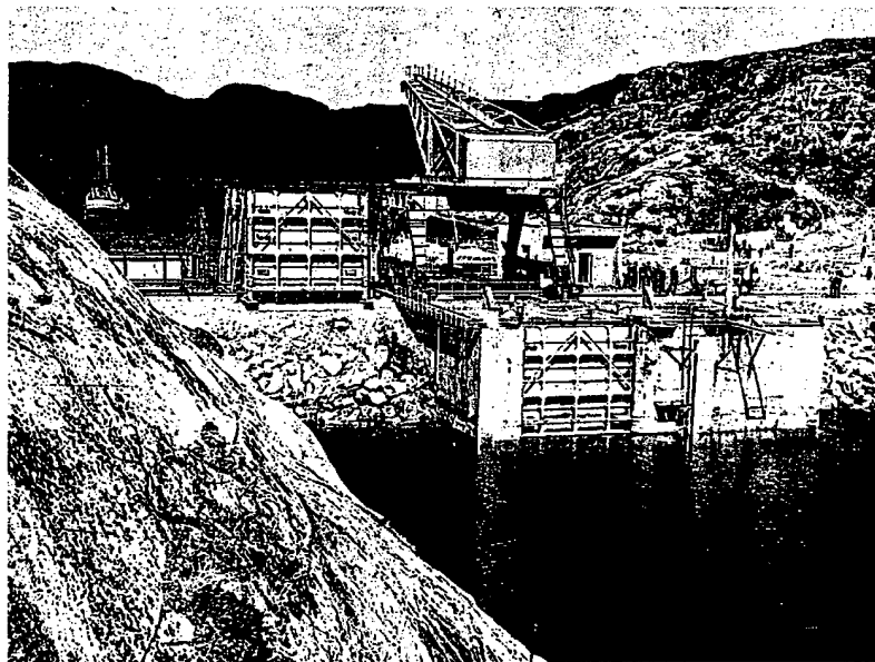
Another view of the Kislaya Guba tidal power station.
