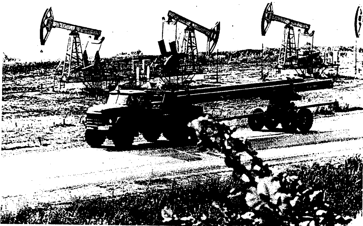
Mechanical pumping units are commonly used to offset low reservoir pressures and lift well fluids.
