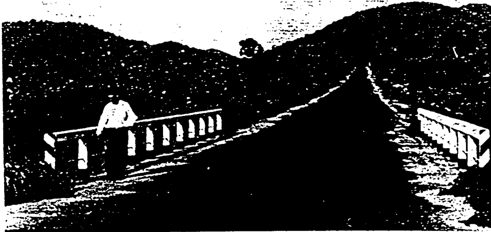
FIGURE 20. Route 11, 7 miles east of Khlong Ngae, Thailand. This main route was constructed as part of the national Six-Year Economic Development Plan (1961-66).
