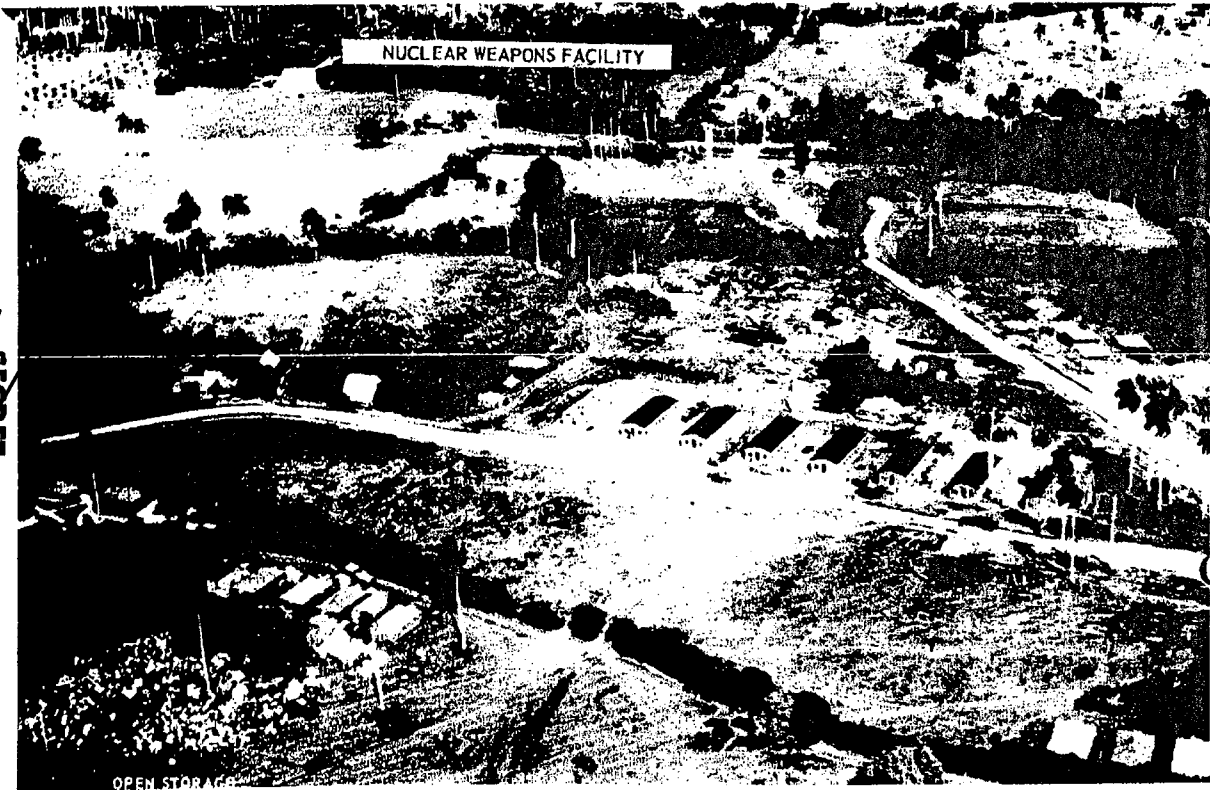
Figure 38. MRBM Launch Site 3 at San Cristobal, 27 October 1962. Construction of permanent support facilities continues.
