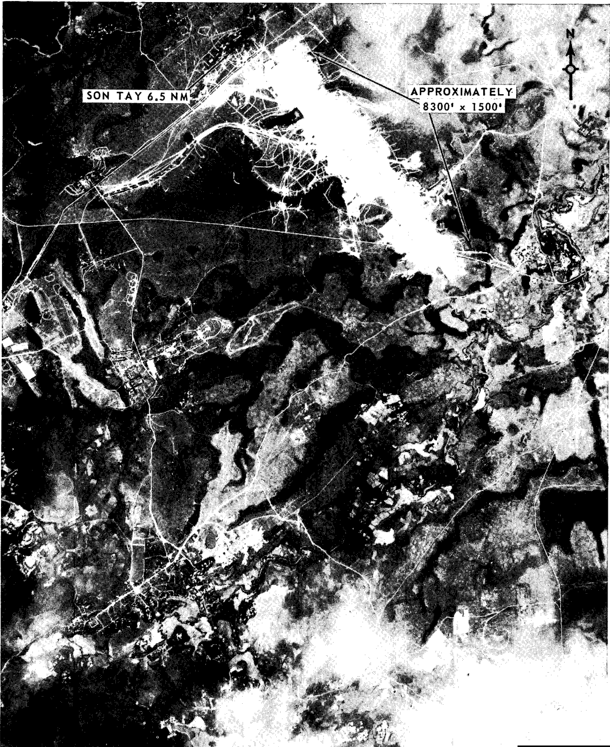
AIRFIELD UNDER CONSTRUCTION, SON TAY, NORTH VIETNAM
