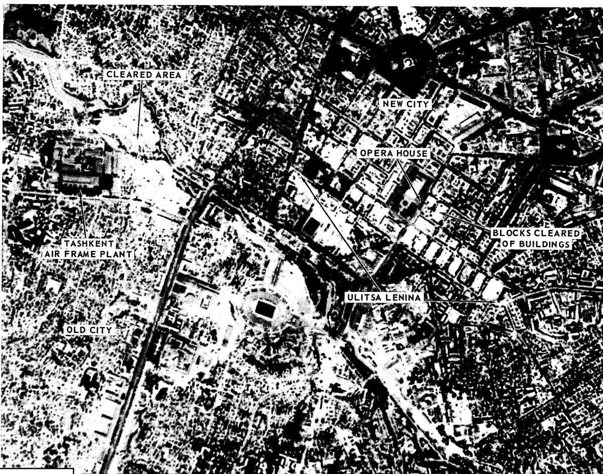
EARTHQUAKE DAMAGE, TASHKENT, USSR
