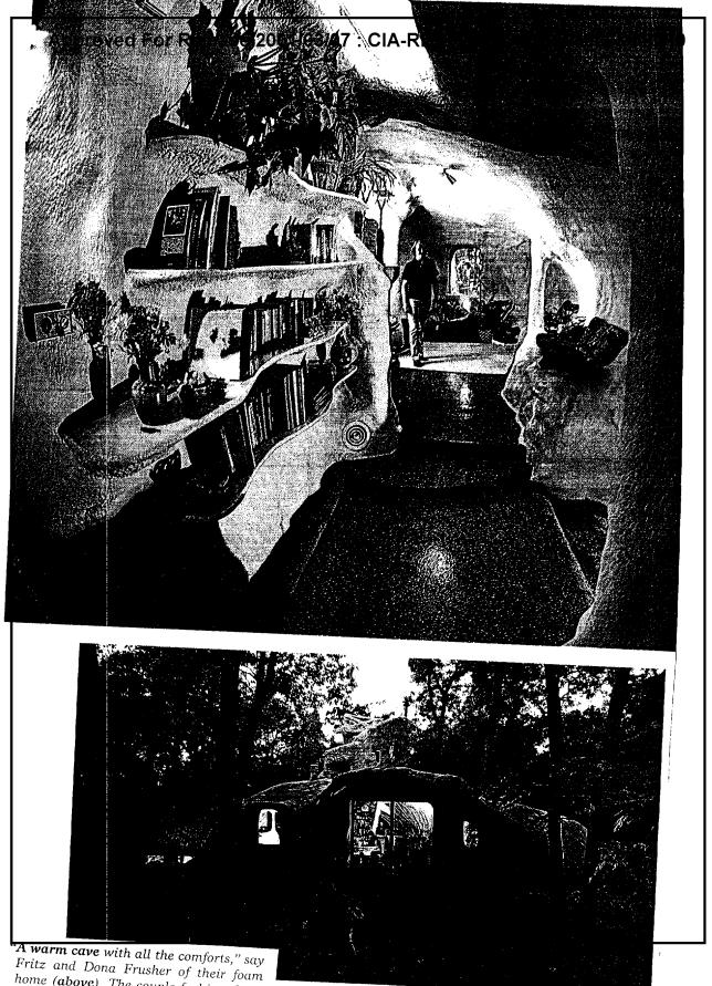
home (above). The couple fashioned the structure by inflating plastic sheets and spraying them, 6 to 8 inches thick, with polyurethane, a material used as insulation. A small forced-air furnace heats the house at a fraction of the cost for a conventional dwelling. The free-form structure seems to melt into its major.
