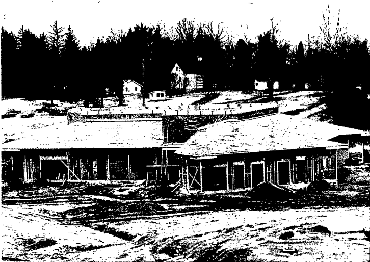
The Agency's Langley Child Care Center nears completion
