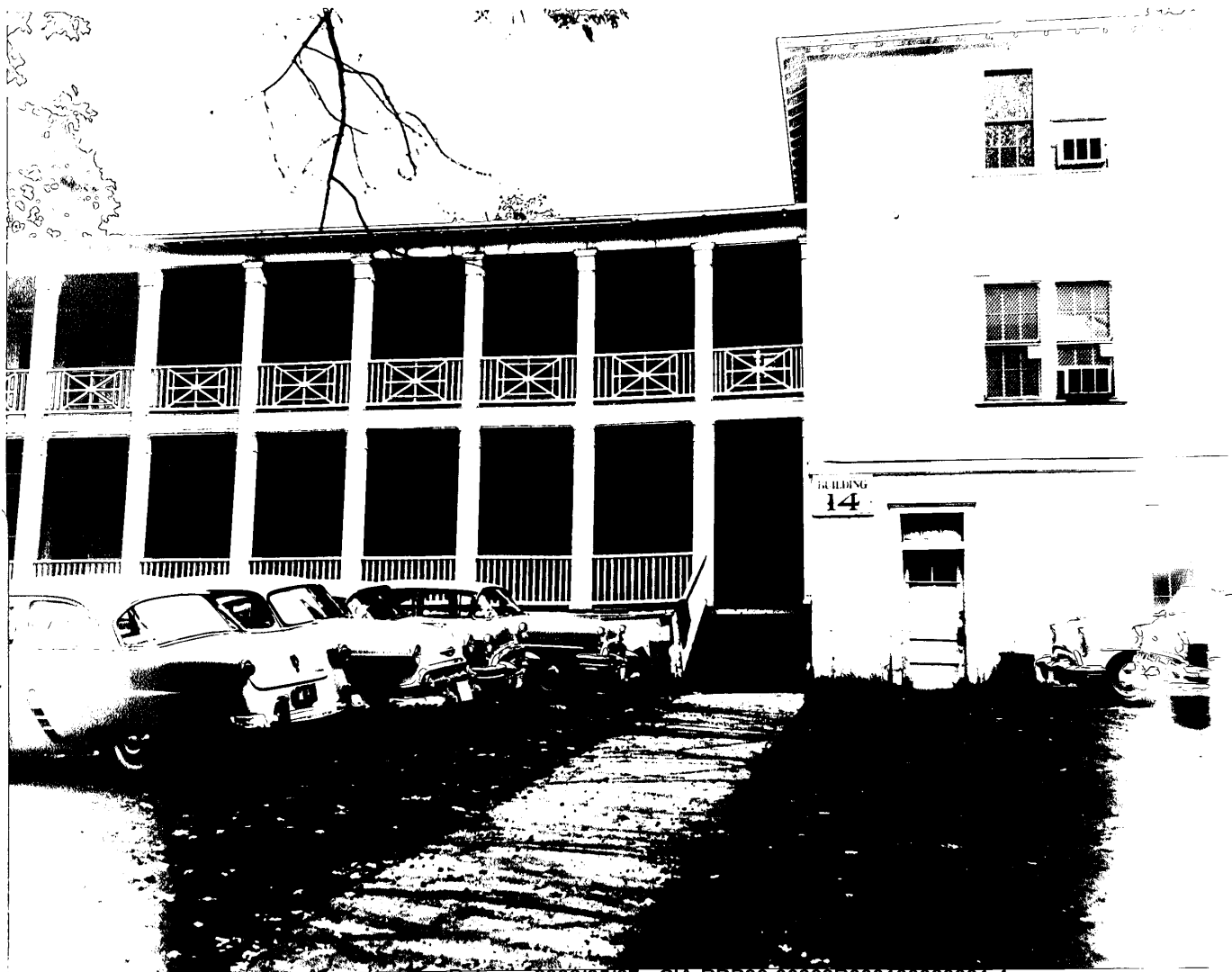
Figure 7 Building 14 (Graphics Register).
