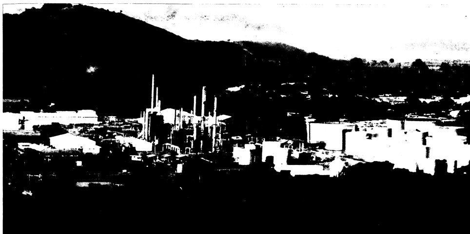
Figure 6. Nicaragua's Only Crude Oil Refinery, Managua. Insufficient repair and maintenance have reduced the facility's output by about one-third.
