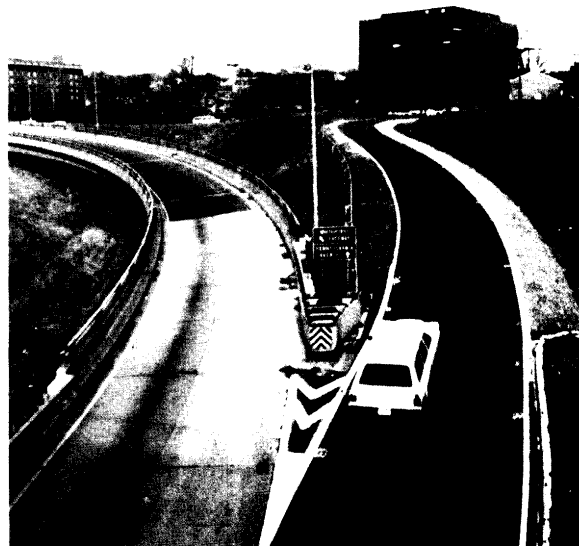
Ramp to the left leading to the Whitehurst Freeway - part of the ramp system addressed in the Whitehurst Freeway Corridor System Modification Study
