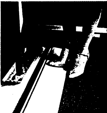
The low profile design of the rail ramp system permits easy passage of foot traffic and wheeled carts.
