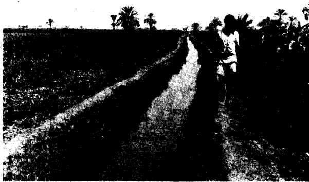
A newly straightened and deepened mesqa (private irrigation ditch) in El-Minya Governorate
