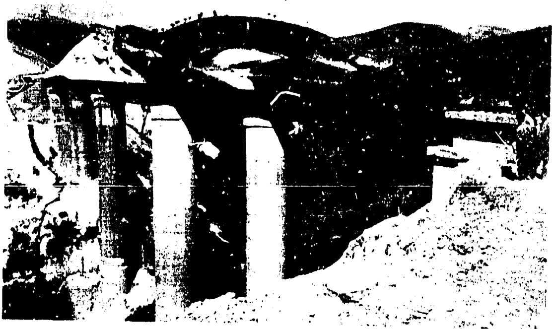
Bridges on the Mlimba-Makumbako section to the Tan-Zam Railroad.
