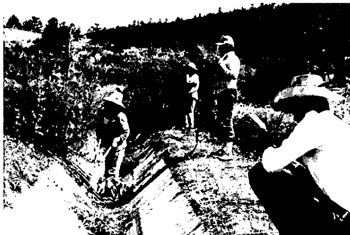
Emergency Jobs Act—funded repair of irrigation ditches on the Confederated Tribe of Warm Spring Reservation, Oregon.
