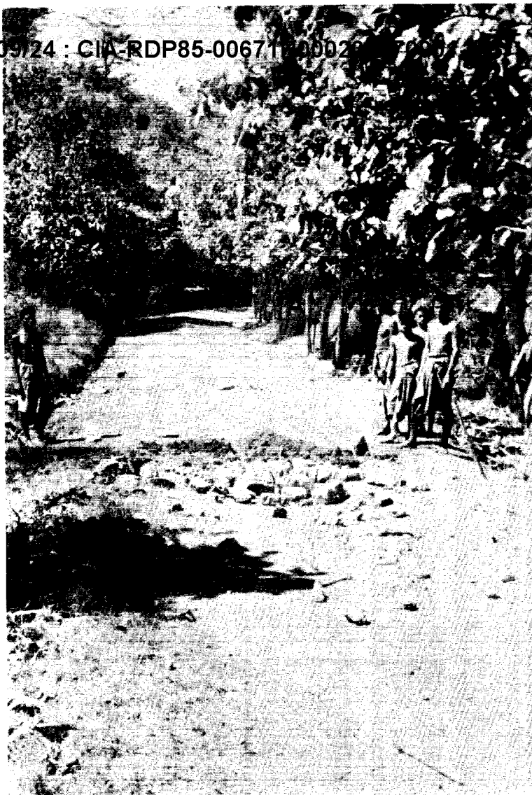
Figure 56. Road main- tenance on road to Ocussi, Timor.
