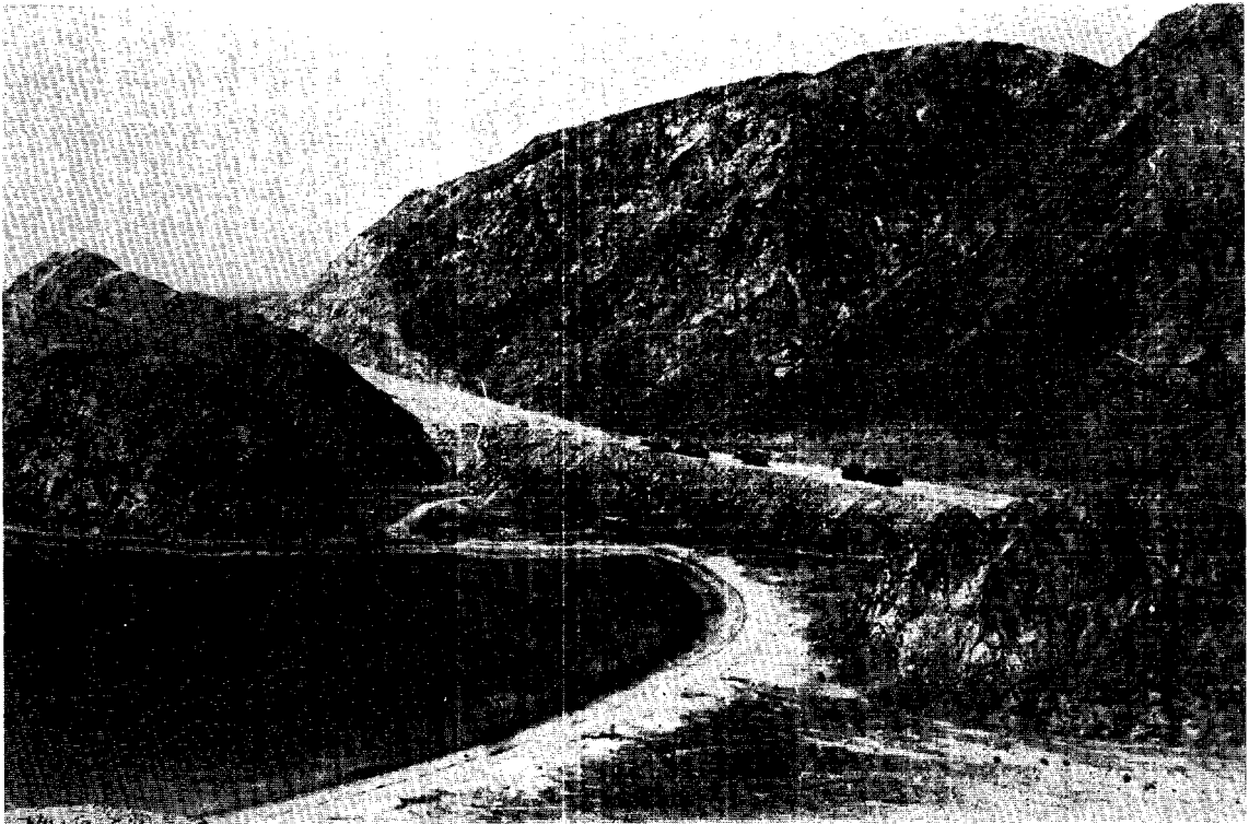
Figure 10. Earthmoving operation on highway from Elat to Sharm ash Shaykh. 10 June 1969.
