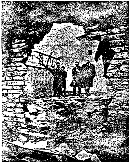
Police inspect blown-out prison wall
