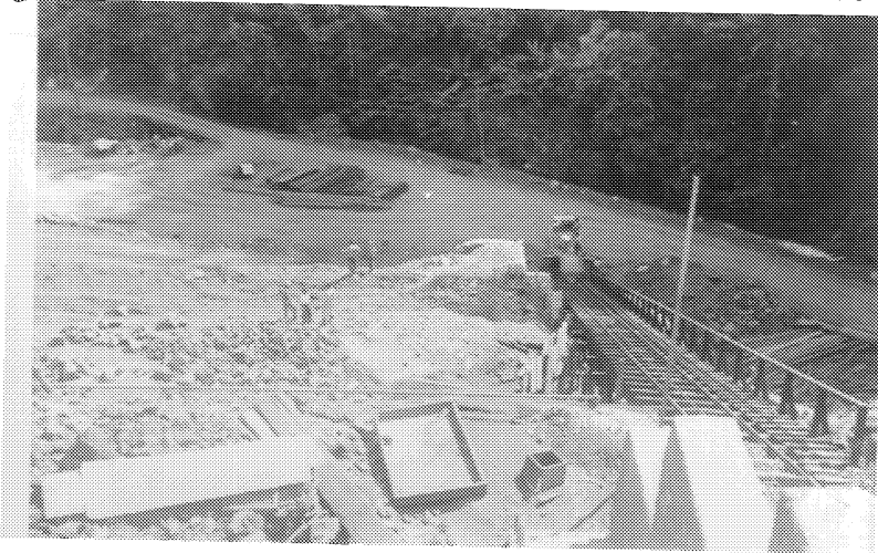
PHILIPPINE ISLANDS MINDANAO ISLAND DAVAO PROVINCE KINGKING 07 09 N 125 54 E CONSTRUCTION 200 TON GOLD TREATMENT MILL OF MASARA MINING Co. FEB.-MARCH 1955. CIA 166723
