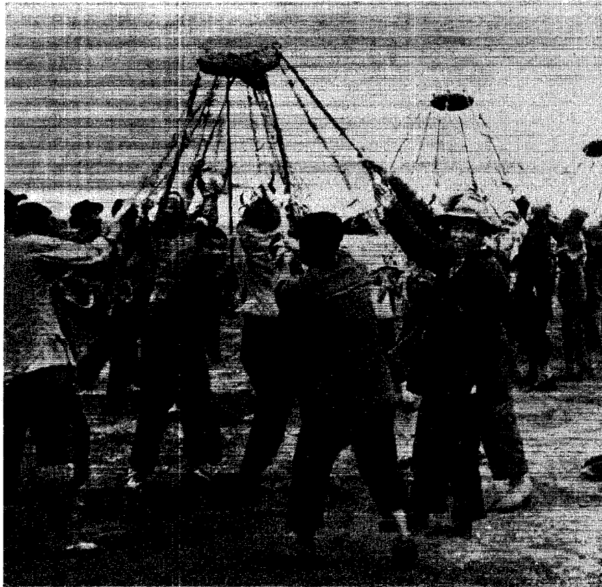
Workers swinging 220-lb. stones to compact earthwork in the traditional Chinese way. Later there will be machines to do this.
