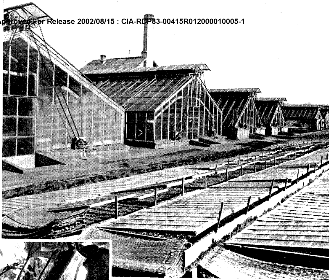
Hot-houses with up-to-date air-conditioning installations
