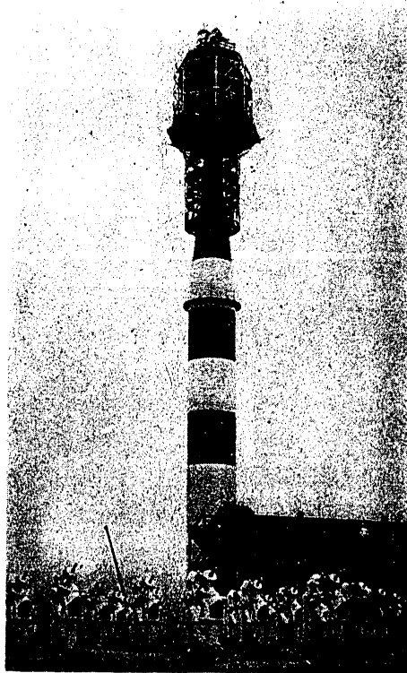
A 1,000 kW Tower Focusing System under construction (Nio-cho, Kanagawa-ken) (p 73)
