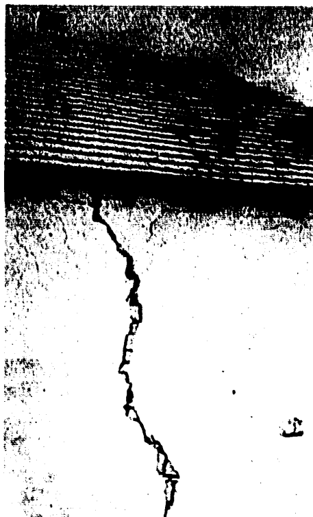
Figure 2. Post Office Building in the Village of Shakhnazar. Cracks in the Walls With "Midis" Masonry
