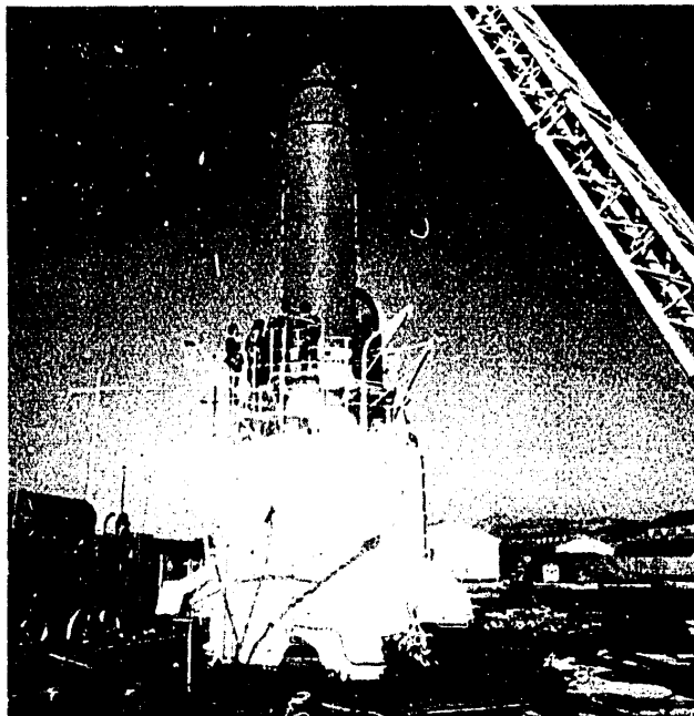
Test mockup of the M4 missile loaded in the tube of the submersible caisson at the CEM [Mediterranean Test Center] in Toulon
