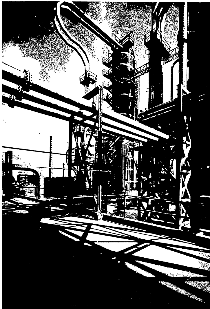
No 1 Ploesti refinery. Part of the atmospheric distillation and vacuum equipment
