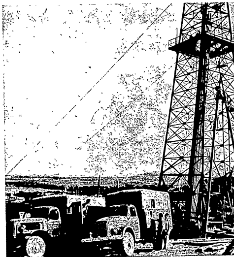
Radio-active logging at a completed well
