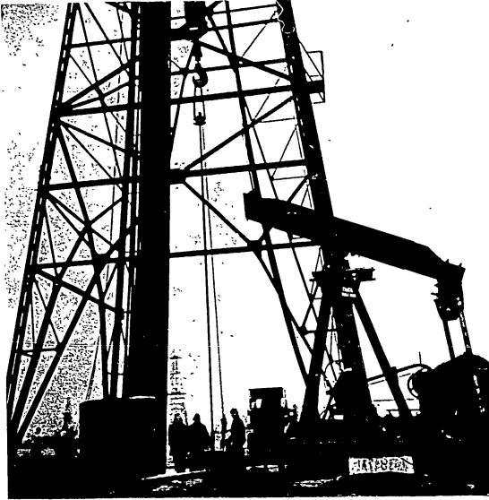
Portable hoist pulling an oil pump on a deep well
