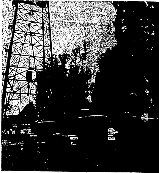
Sliding a metal derrick from one location to another without dismantling
