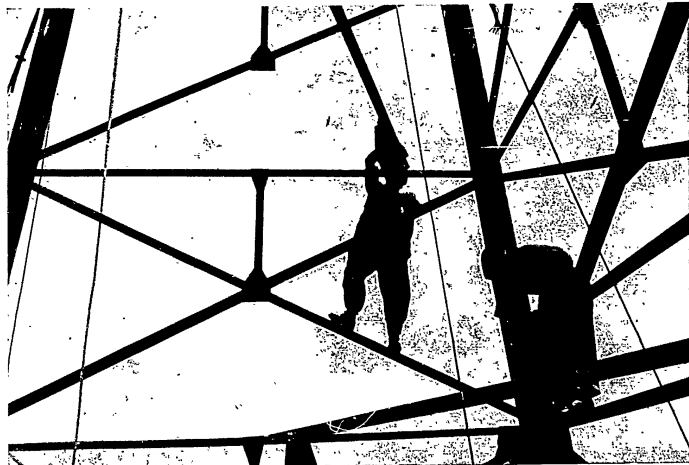
Mounting a metal derrick
