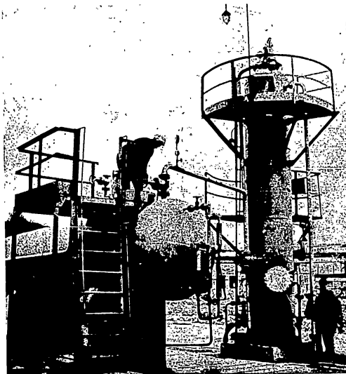
Kerosene-neutralizing equipment at No. 8 refinery in Moldavia
