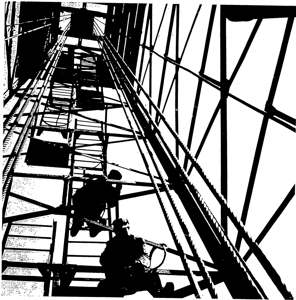
Inside view of a steel derrick
