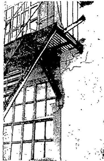
Wall Deformed by a Rigidly Joined Fire Escape Heaved by its Shallow Foundation.
