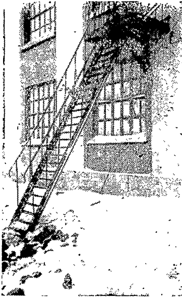
Wall Deformed by a Rigidly Joined Fire Escape Heaved by its Shallow Foundation.
