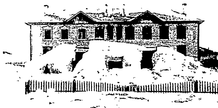
Snowdrift on Lee Side of a Building Erected at Right Angles to Prevailing Wind
