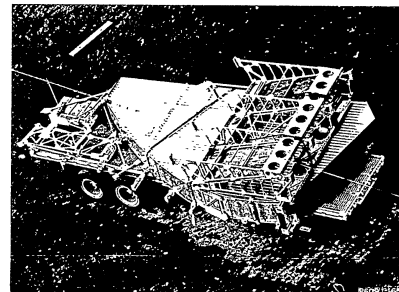
Fig. 71-22. Hog horn, upper supports, rear support and pivot arms as shipped from the fabricator required special road escorts because of 15-foot width.
