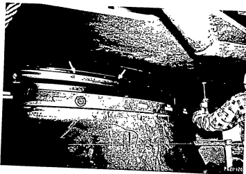
Fig. 71-28. One of the guide pins accurately locating the hub before it was finally lowered into the bearing by the jacks, one of which can be seen being operated. The arrows show a chatter mark on the bearing pilot diameter of the hub. This in no way affected the bearing quality or installation.
