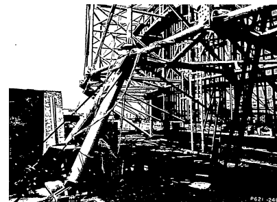
Fig. 71-2. Reflector rear support leg showing strain gage wiring terminating of instrument panel.
