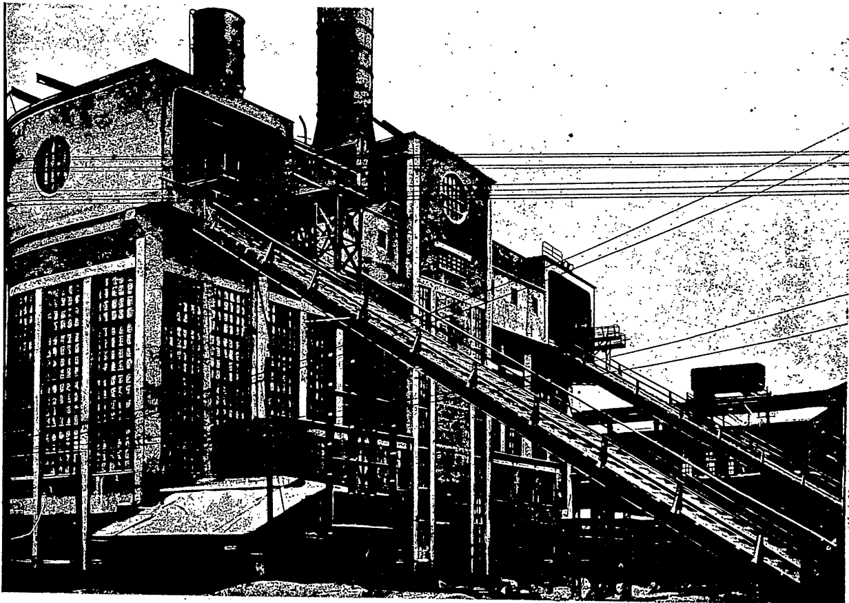
Side view of the boiler house.
