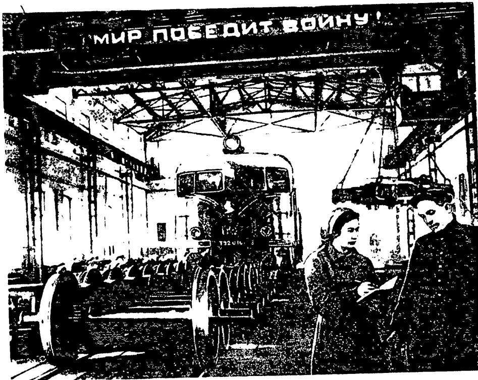
Fig. 21 - Running gear repair shop of Chelkar enginehouse of Orenburg System.
