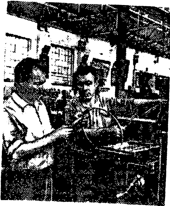
Fig. 12 - At preliminary-processing shop of Tashkent-Freight diesel locomotive enginehouse.
