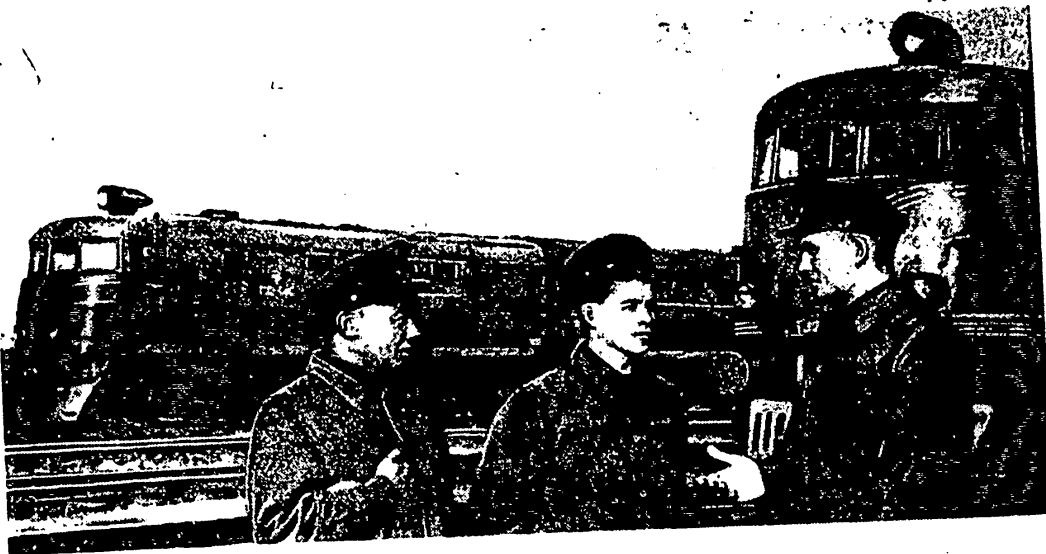
Fig. 19 - Diesel locomotives on tracks near Chelkar enginehouse of Orenburg System.
