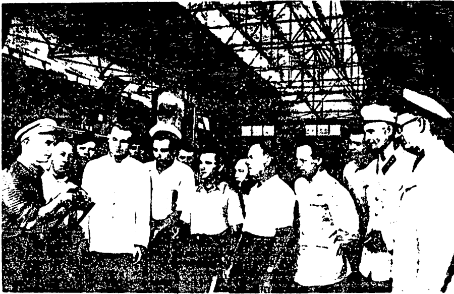
Fig. 10 - At Tashkent-freight diesel locomotive enginehouse.
