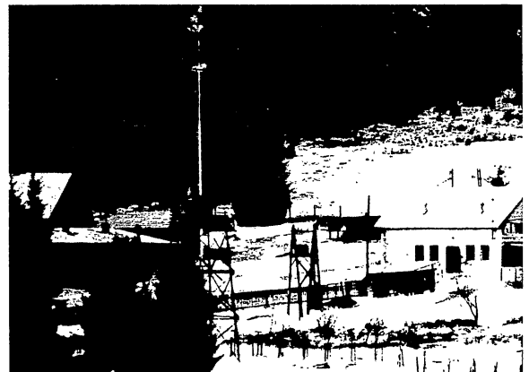
A TYPICAL COMPANY AREA WITH A TRANSFORMER TO THE RIGHT REAR OF THE OBSERVATION TOWER
