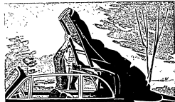
Draft and dust-free sealing of the hard-wearing top. Closing of the top can be performed with very little physical effort. The side windows drop flush.
