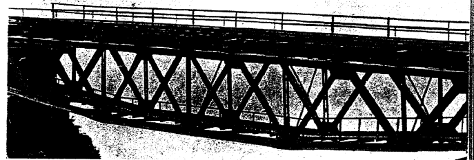
1022 A model of the bridge across the river Váh, at Púchov, Czechoslovakia Welded throughout. Length 187 metres
