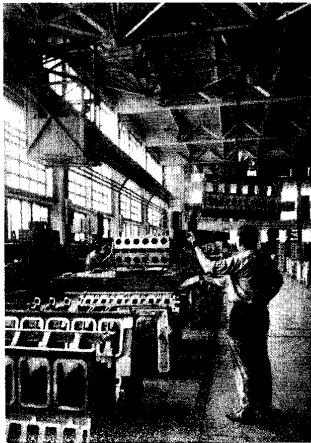
Assembly of a diesel engine, several hundreds of which are manufactured yearly to power various types of rolling stock.
