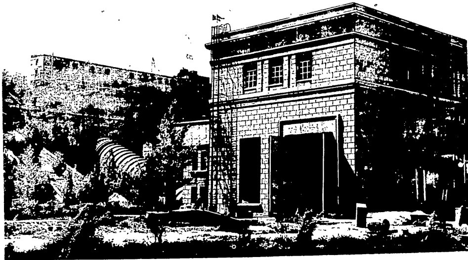
Fig.4 Farkhad hydropower plant
