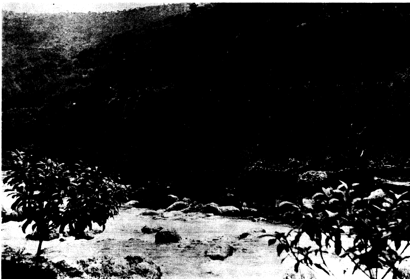
Canal, leading from Jeita Spring to the Hrach Power Plant.
