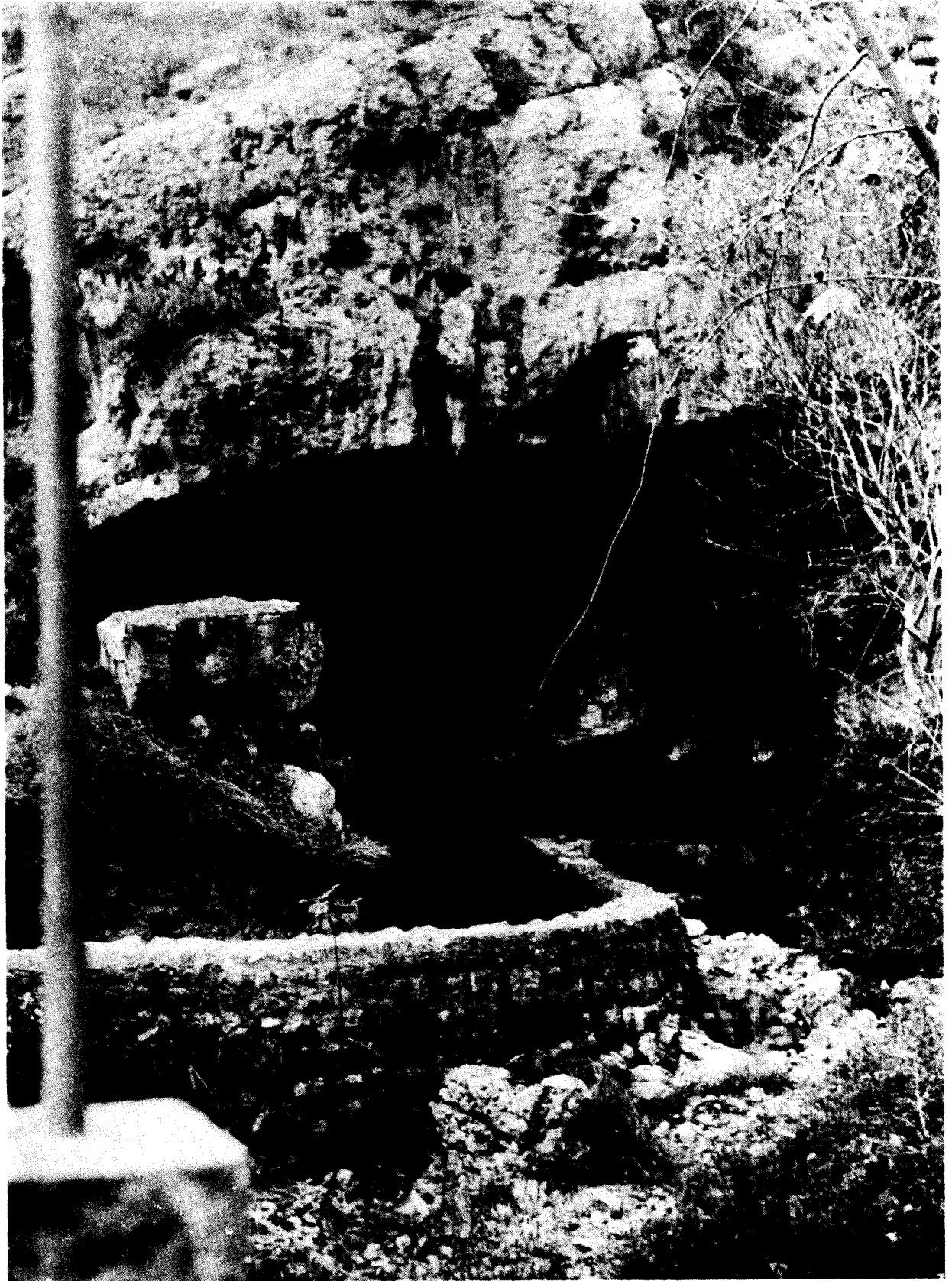
Jeita Spring and Inlet of Canal leading to the Hrach Power Plant.
