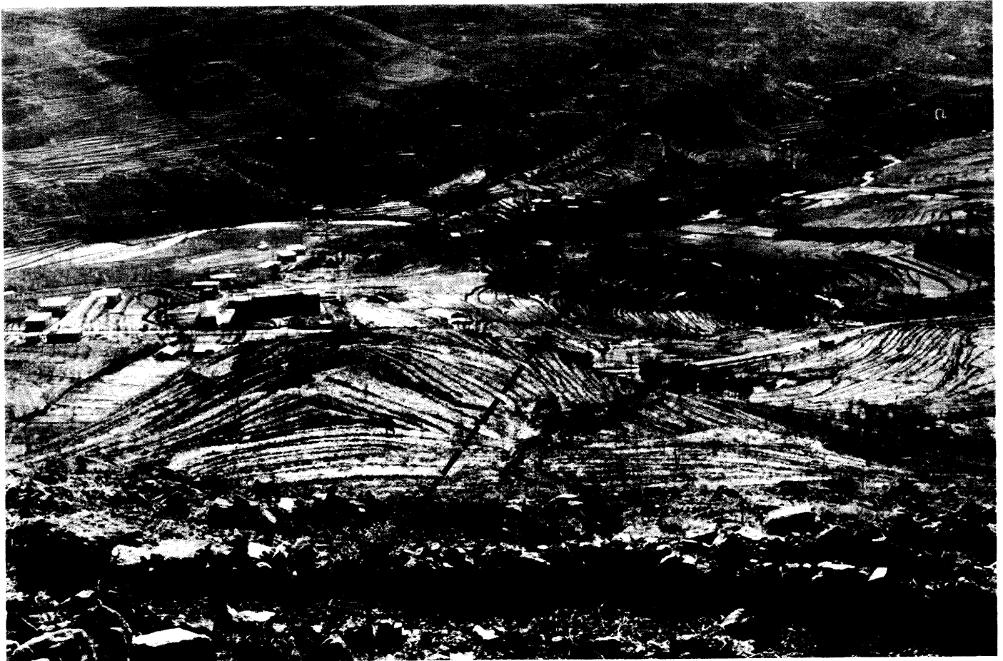
Hardoun Penstock Lower section of penstock alignment. The upper end of the Mayrouba reservoir would occupy the valley in the distance.
