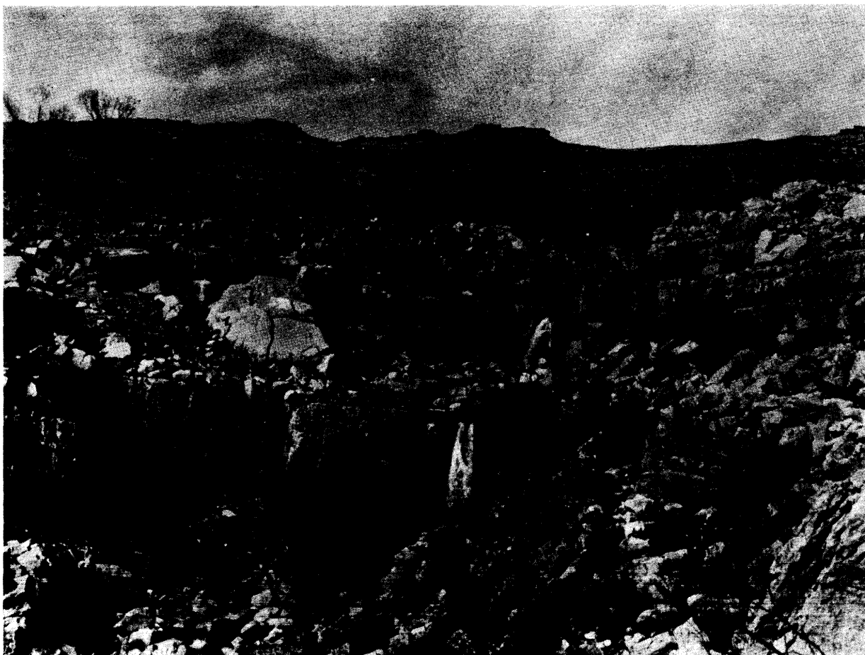
Hardoun Diversion Dam Site Talus obscures the foundation for this structure located at the edge of the pool below the lower falls.
