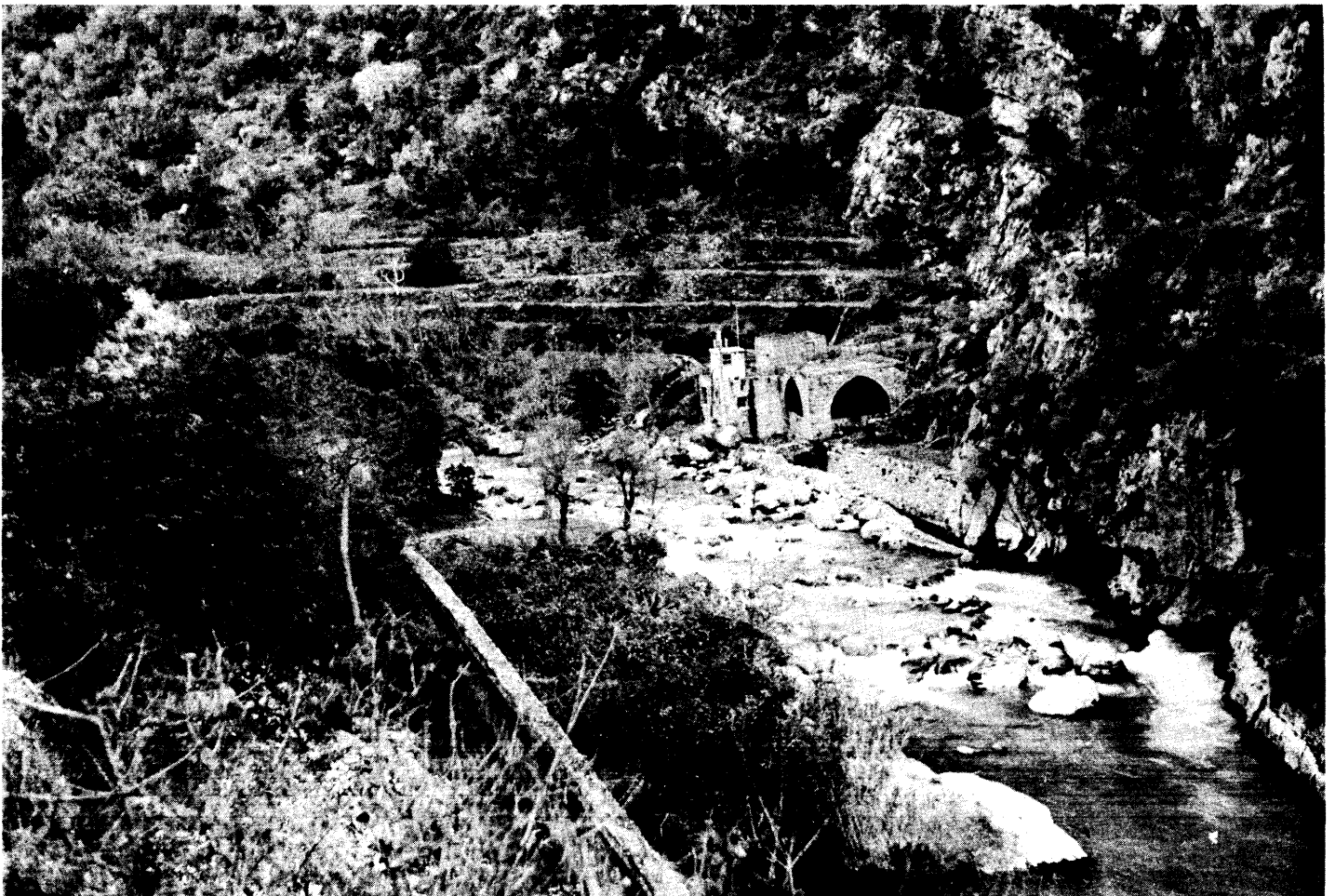
Tahoun el-Khoury Power Plant
