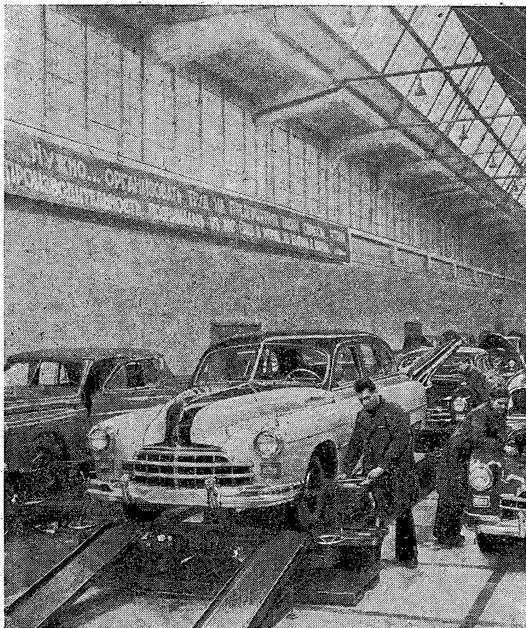
Assembling ZIM passenger cars at the Molotov Auto Plant in Gorky
