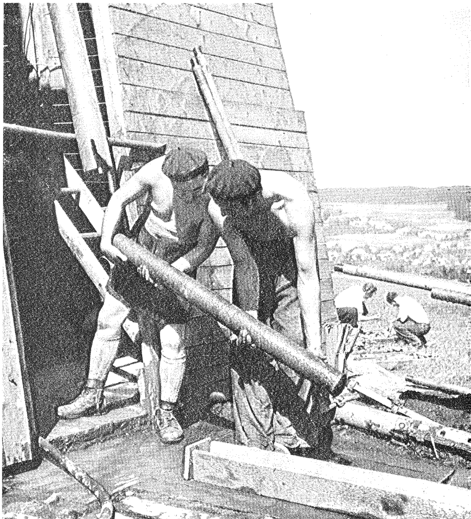
We are finding new raw materials for our industry. This portable boring installation is used by our geologists who also research on mineral ores and dam construction.
