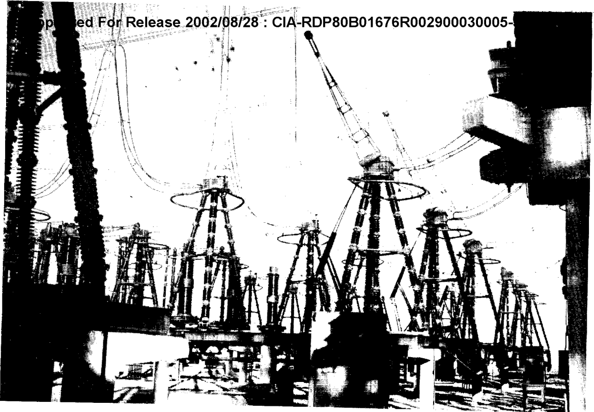
Figure 19 - 500 KV Disconnect Switches
