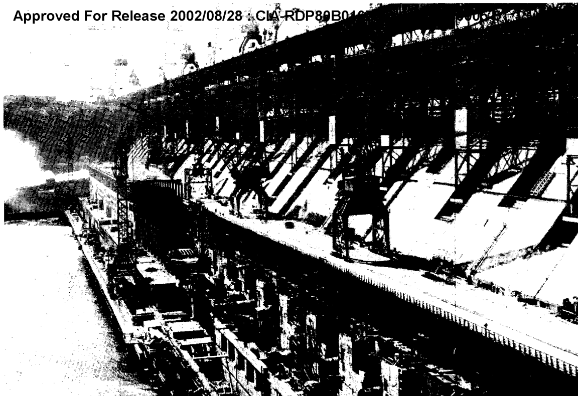
Figure 5 - Downstream portion of Bratsk Dam
