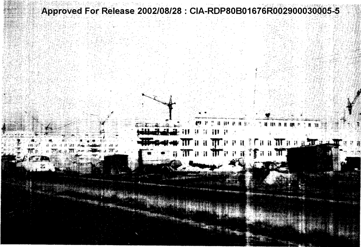
Figure 44 - Apartments under construction. Housing like this is part of the scheme of having workers live near the factories they work in. The apartment houses are made of precast concrete
