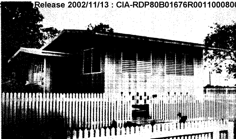
A TWO-BEDROOM BUNGALOW, the smallest of the several types of houses to be constructed on the 600-house, 110 acres site on Highway 54, Quezon City. Shown is one of the first four model houses. Three hundred houses were scheduled for completion by November, 1954 and the additional 300 homes are scheduled for early 1955.
