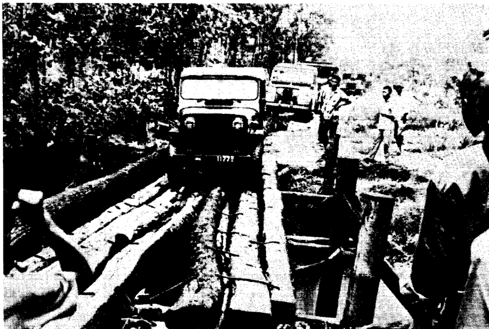
Figure 11. Rickety bridge on secondary road between Route 13 and Siem Pang.
