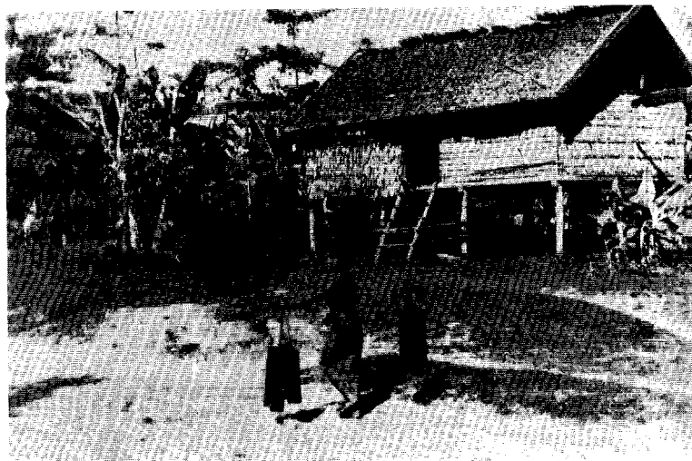
Figure 7. Khmer peasant house of bamboo and palm frond construction.
