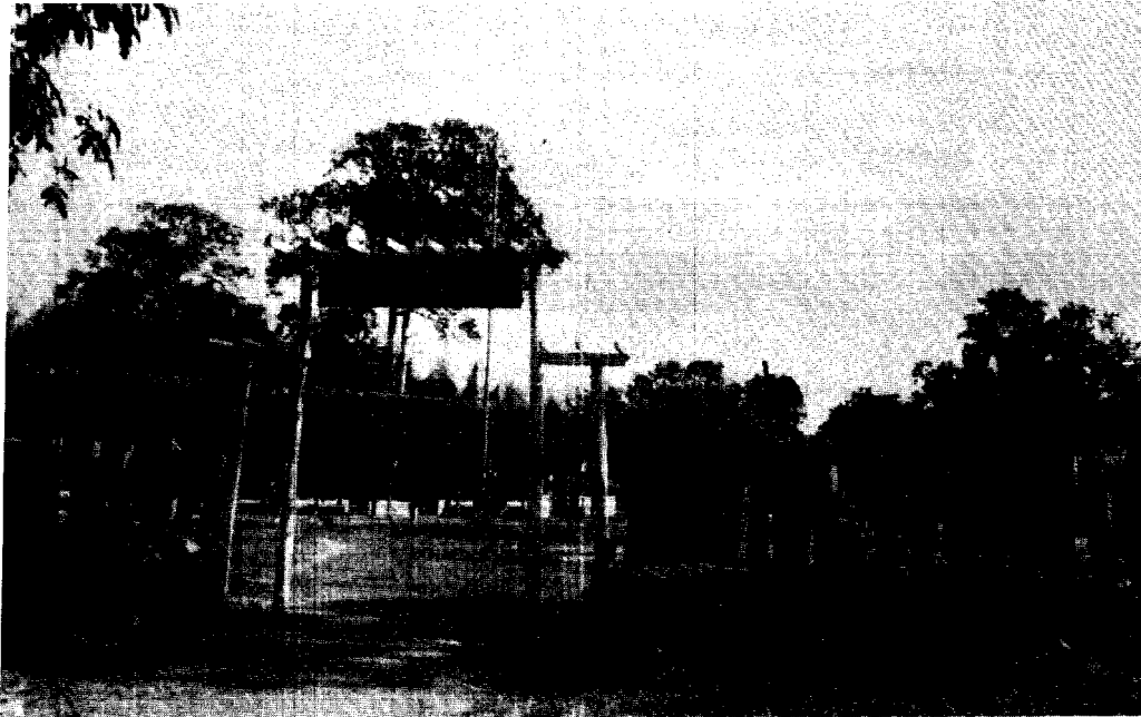
Figure 14. Provincial Guard post. April 1966.
