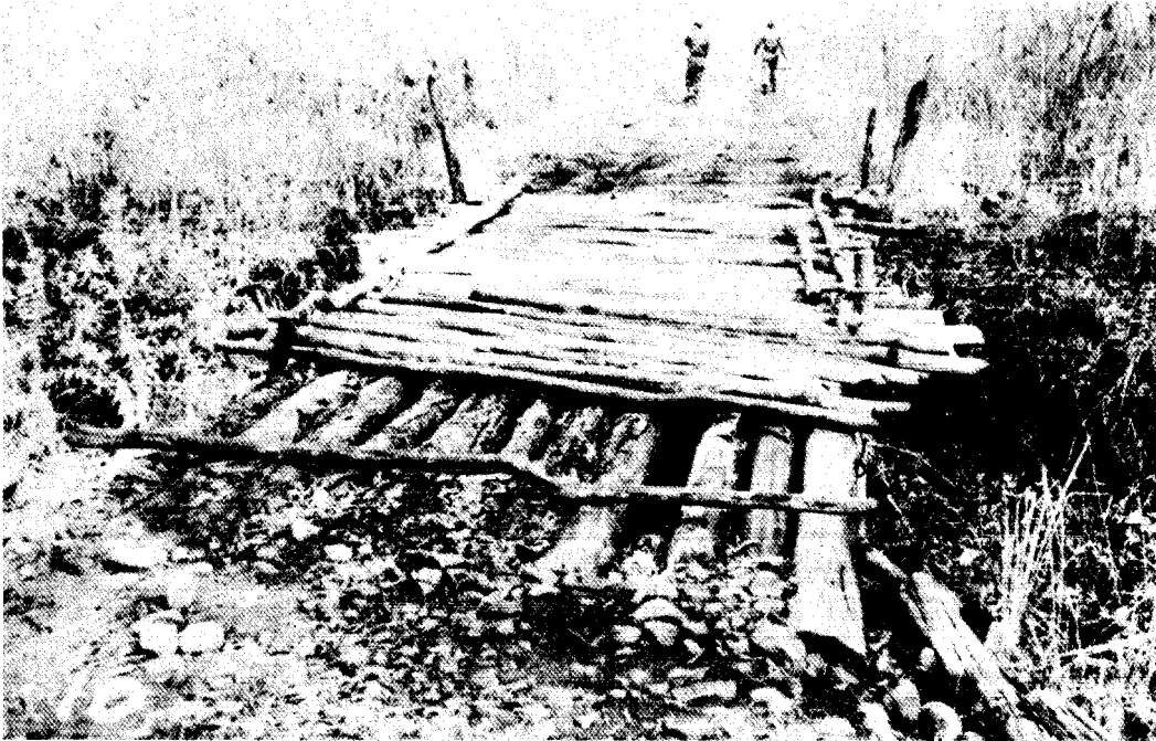
Figure 12. Makeshift bridge along secondary road near Poste Deshayes in Mondolkiri Province.
