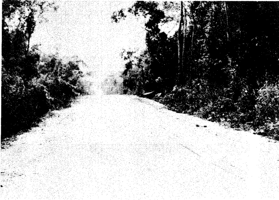
Figure 4. Graded earthen road on plain north of Tonle Sap.
