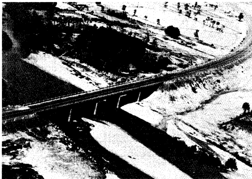
Figure 13. Bridge on Khmer-American Friendship Highway near Kompong Speu.
