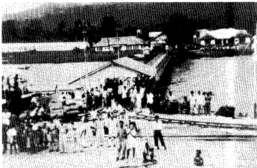
Figures 156 & 157. Two views of pier in Ternate harbor. Expansion of port facilities was begun in 1964, after these photographs were taken.
