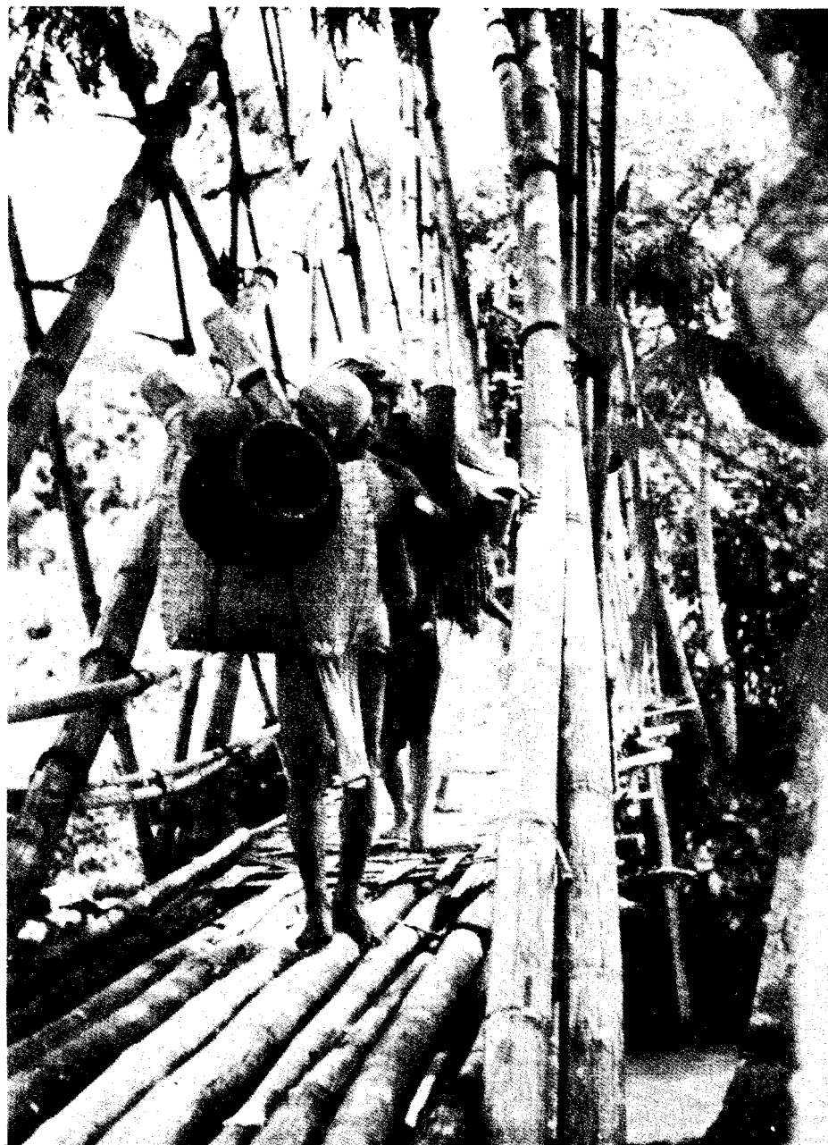
Figure 149. Bamboo footbridge on Celebes. Such bridges are commonly washed away by flash floods.
