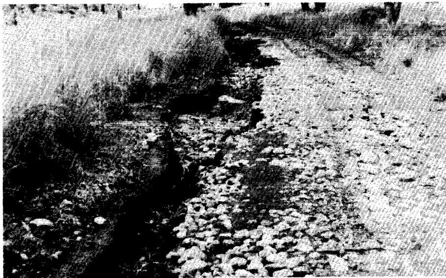
Figures 132 & 133. Main east-west road on Flores. Note rapidly encroaching vegetation in upper photo, which has nearly engulfed road. Muddy condition would preclude use of road by most vehicles in wet weather. Lower photo shows typical washout due to inadequate drainage. 1959
