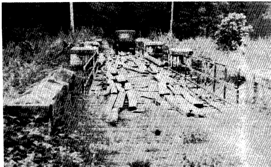
Figures 134 & 135. Bridges on main east-west road on Flores. Condition of bridge floors is typical. 1959
