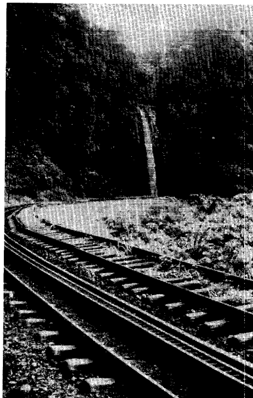
Figure 58. Rack section on railroad north of Lake Singkarak ( 00^{\circ} 37'S-100^{\circ}33'E ). Such systems are necessary to ascend steep slopes.
