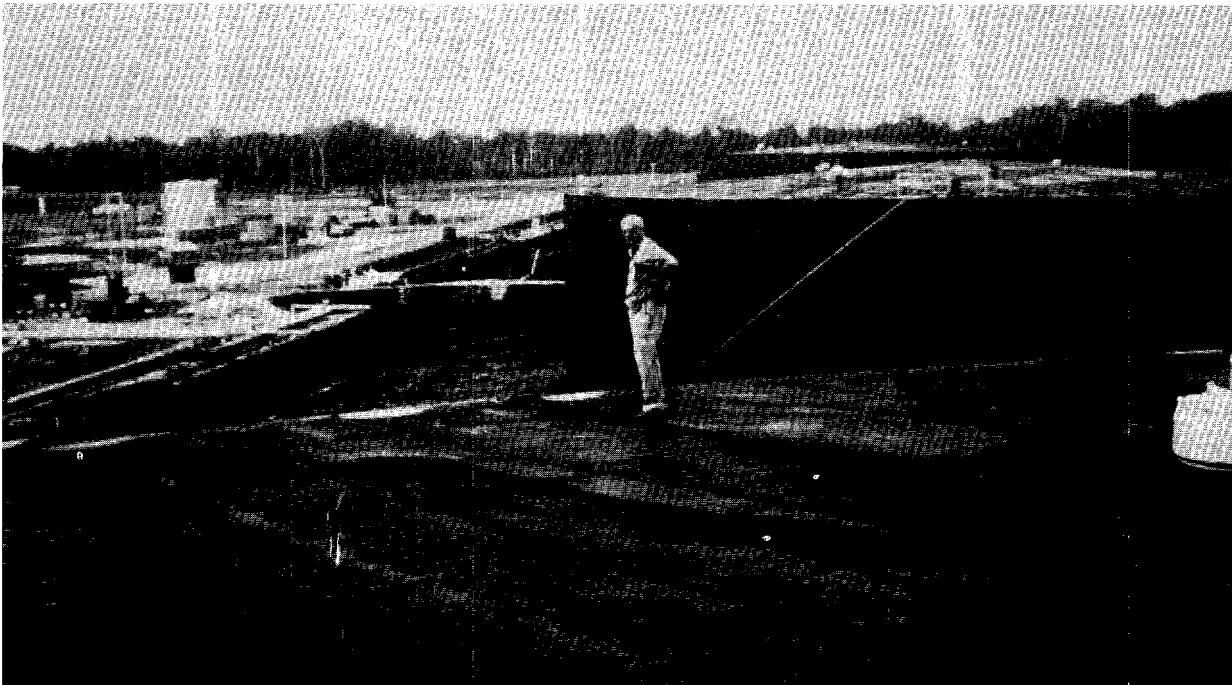
Figures 44 and 45. Oil pumping station at Dumai. New Caltex tanks under construction (June 1964).
