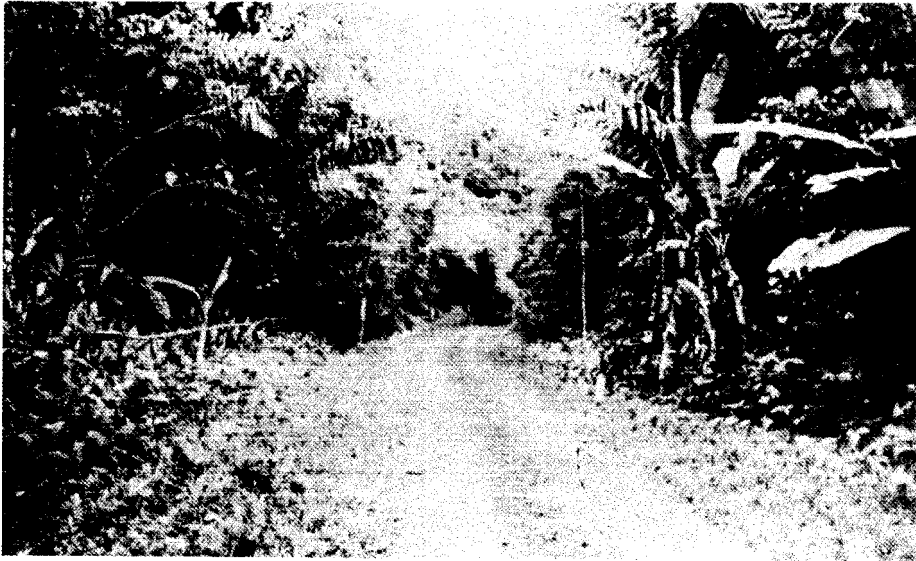
Figure 49. Gravel-surfaced road, illustrating problem of encroaching vegetation.
