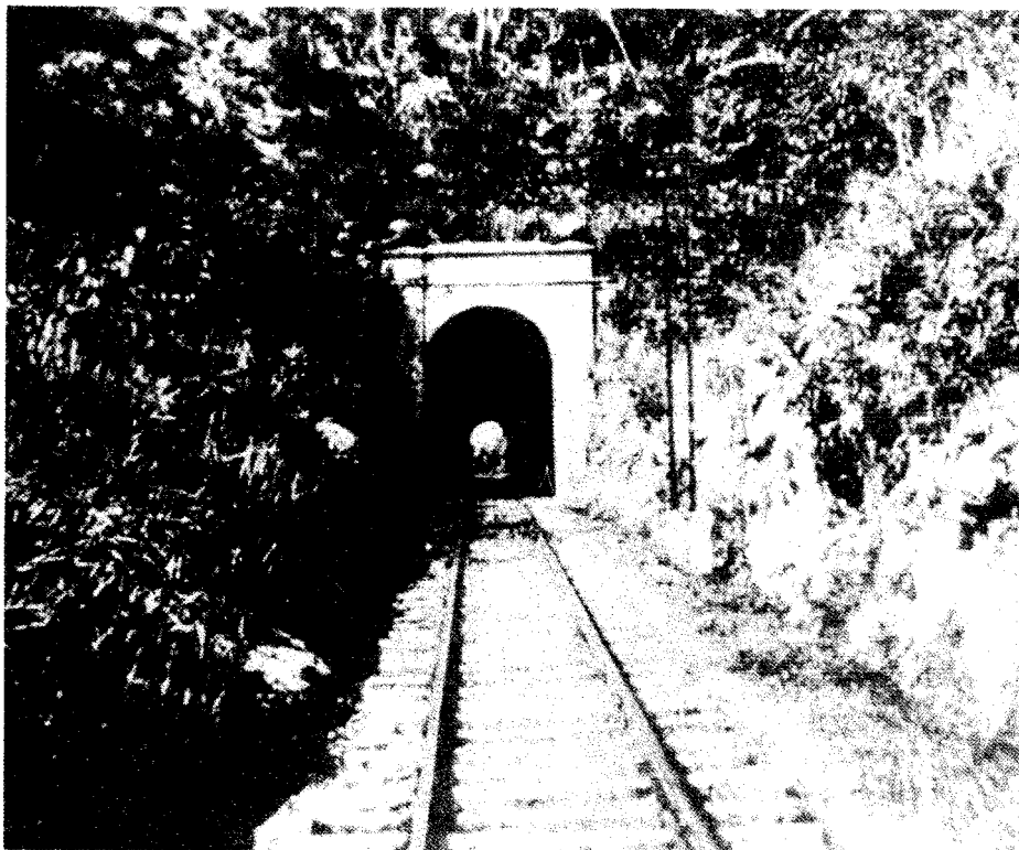
Figure 53. Pangalat Tunnel, on the railroad, located 3.3 miles northeast of Papar ( 5^{\circ}45'N-115^{\circ}58'E ). This tunnel is 600 feet long.
