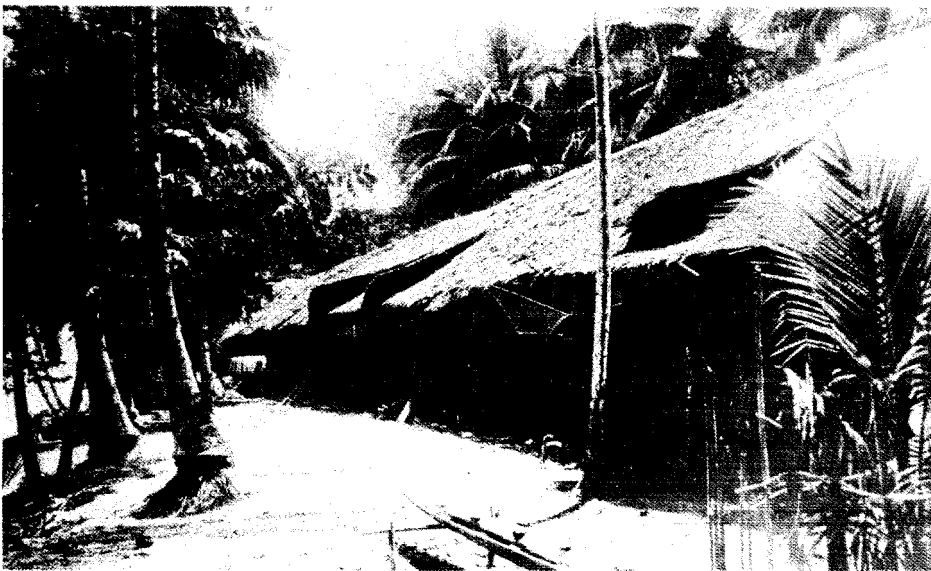
Figure 35. A Murut longhouse. Sections of the roof are propped open to admit light to the family compartments. Communal houses are being replaced among the Muruts by smaller dwellings.
