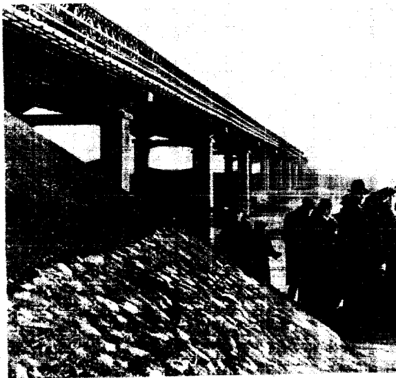
A newly constructed bridge across the Vistula in Pultusk.
