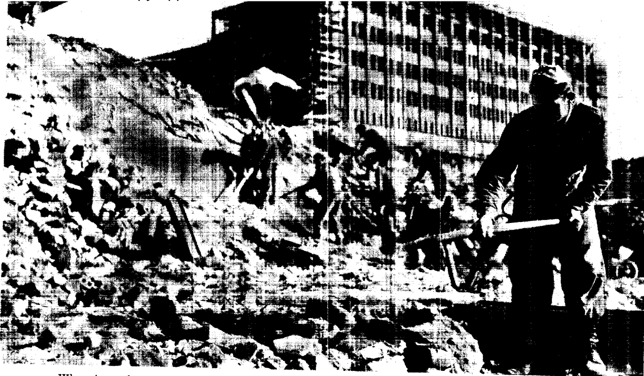
When in a place the ruins are still being removed, mighty buildings are already being constructed.
