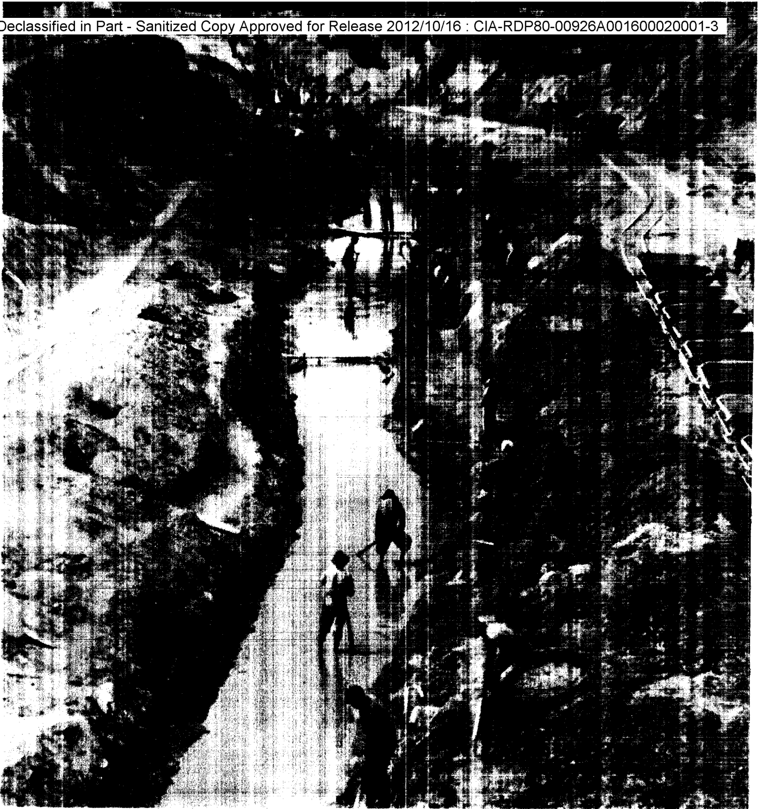
Co-operation between town and countryside was resulted in the building of new irrigation canals, and consequently, watering and drainage for the land. The Danube-Tisza canal under construction.
