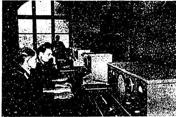
Fig. 7 — Police Radio Communication Headquarter in a Large City.
