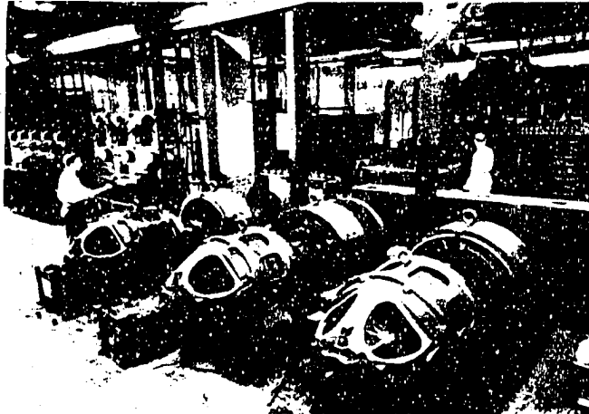
Fig. 1 - View of the miniature replica system used to investigate the effect of charging kva on steady state power limits.
