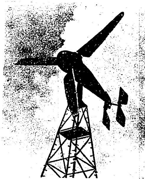
Fig. 4 — Porsche 10 kW wind power plant of 9.2 m diameter, 1944.
