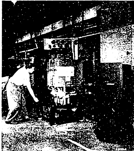
Fig. 7 — 15 kV circuit breaker withdrawn from metal clad switchgear and covers removed. benefited by the ease with which breakers may be interchanged during inspection procedures. Components, such as current transformers and bus, Figure 8, are readily reached for inspection, maintenance or extension. Removable coverplates and barriers provide access to these components. Potential transformers may be withdrawn to a de-energized and grounded position for inspection and replacement of fuses.
