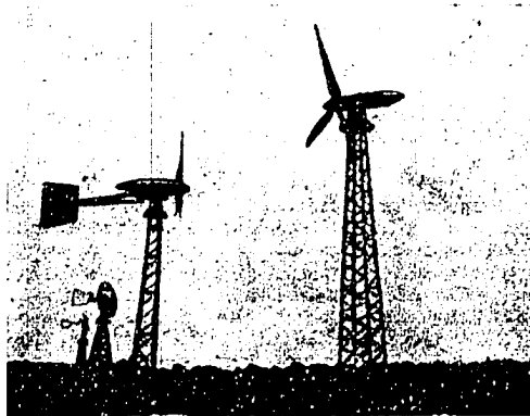
Fig. 3 — Test field of Ventimotor G.m.b.H. Weimar 1943. From right to left: 10 kW D.C. plant of 10 m diameter with fully electric control, 50 kW plant of 18 m diameter with mechanical control, "Stahlwind" plant of 7.2 m diameter for parallel operation tests, "Koster" wind-driven pump of 7 m diameter.
