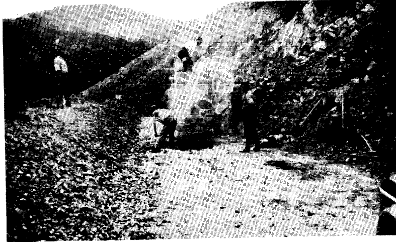
Figure 9. Local workmen using mobile rock crusher. Small crushers of this sort are moved from village to village and are used to prepare material for both the improvement and the maintenance of roads.
