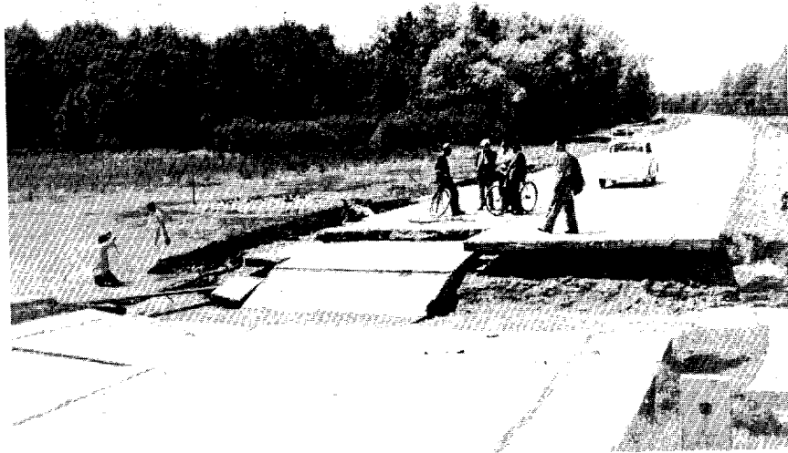
Figure 3. The highway between Belgrade and Zagreb after a flood. Although this is the best highway in Yugoslavia, it is subject to serious flood damage.
