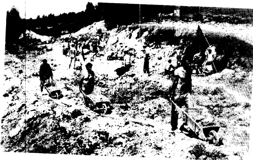
Figure 7. Youth Brigade at work on the Ljubljana-Zagreb superhighway. Much of the cutting and filling on this road project was done by manual laborers of such brigades.
