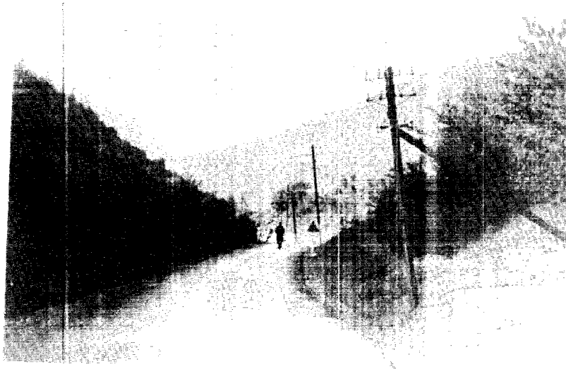
Figure 4. Part of the first-class route between Split and Sarajevo. Most of the road is narrow and has developed a washboard surface.
