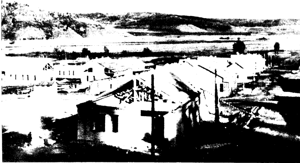
Figure 9. Oilfield workers' settlement under construction in the Zhiguli Mountains near Kuybyshev.
