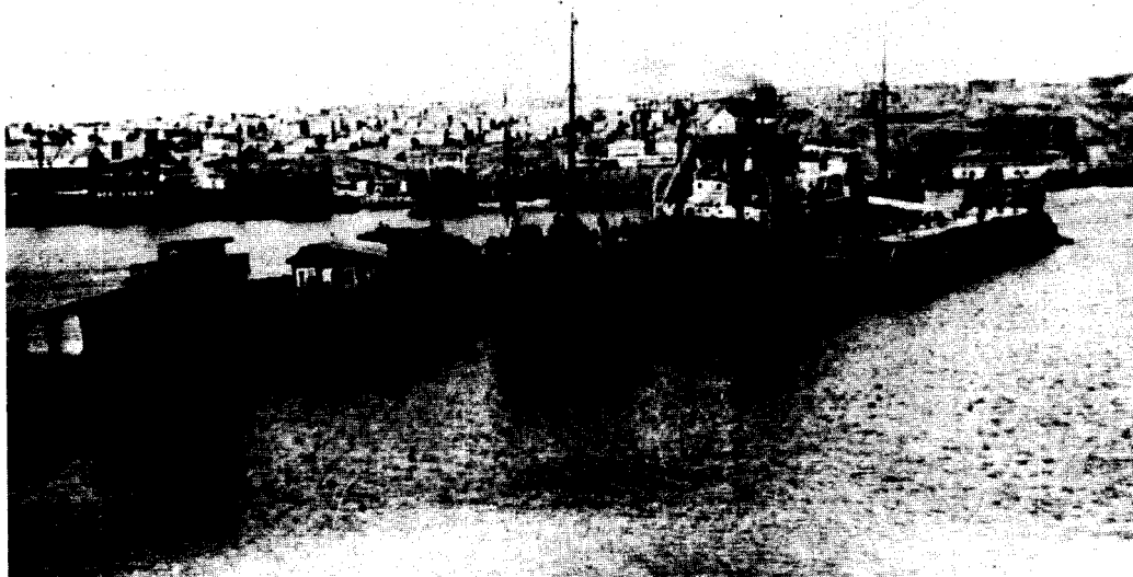
Figure 5. Freighters at anchor in Igarka.
