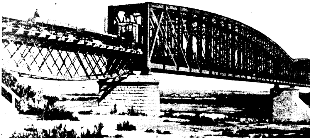
Figure 46. Bridge over the Ishim River west of Petropavlovsk.
