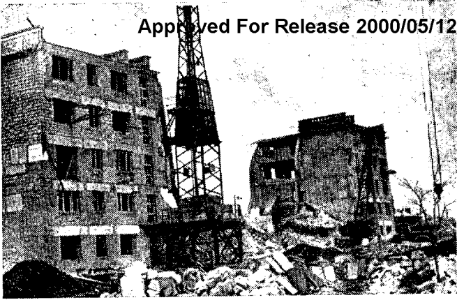
The structural failure at Odessa
