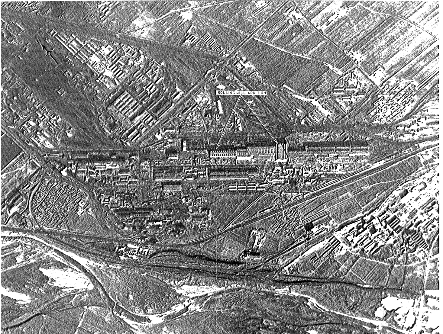
FIGURE 14. SHIH-CHING-SHAN IRON AND STEEL PLANT.
