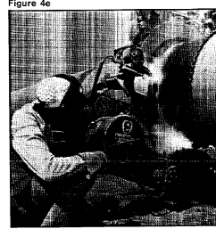
Figure 4e Final Pipeline Arc Welding Operations
