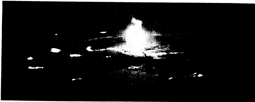
Figure 5. Dramatic night shot of Panarctic's burning gas well on King Christian Island in the Canadian Arctic, showing both the 150-foot high flame from the well bore and a number of fissures in the ground, with gas escaping and burning 1,000 feet or more from the collapsed drilling rig.
