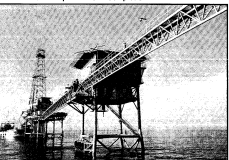
Figure 1. Standard Triple-Platform Completion
