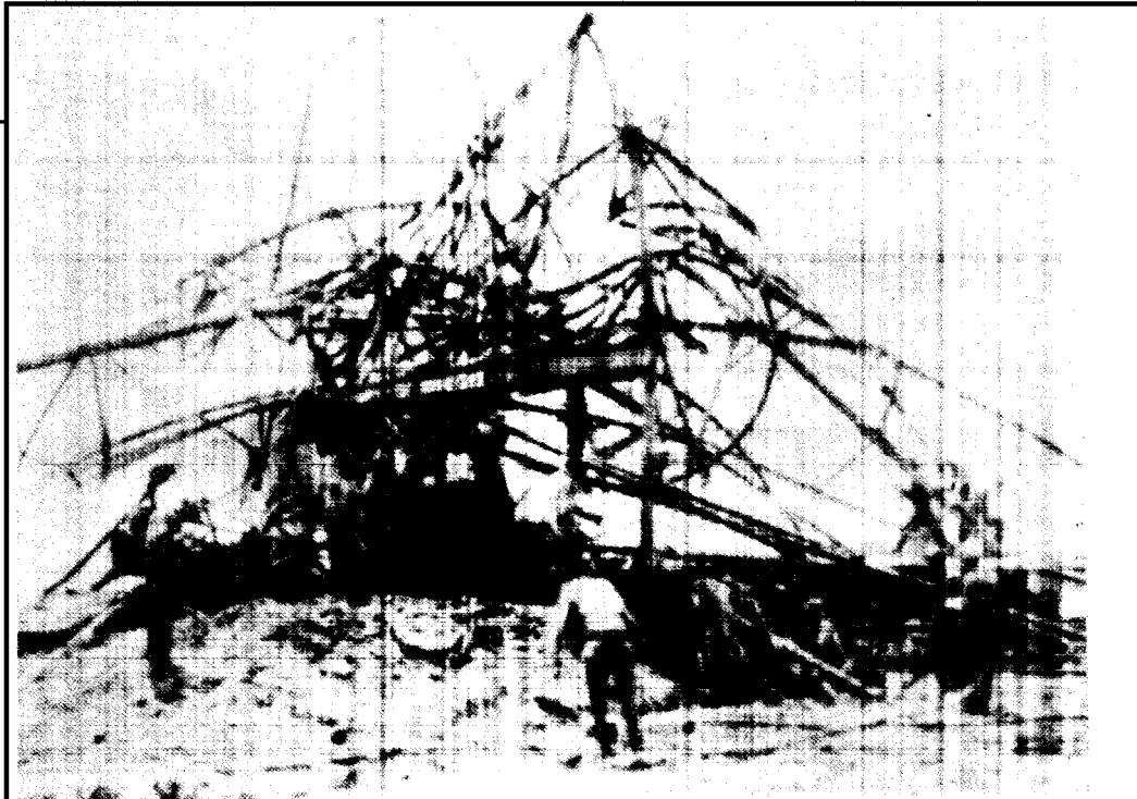
Figure 3. BLOWOUTS ON ROTARY WELLS occurred frequently in the early days. This rig was almost demolished.
