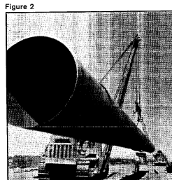
Figure 2 Pipe Stringing and Offloading along Right-of-Way
