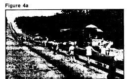
Figure 4a Pipe Alignment, Joining, and Welding Operations
